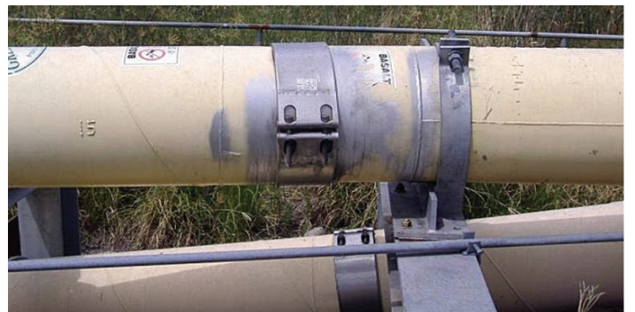
MJS EPDM 400A. mineral conveying line. Australia
