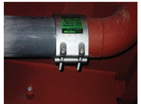
MJS EPDM 100A. PVC pipe + steel pipe. Korea
