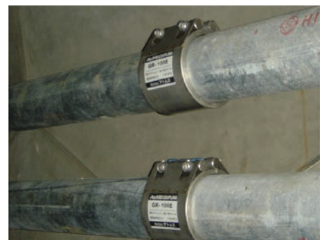
MJGF EPDM 100A, drain pipe, subway station, Japan
