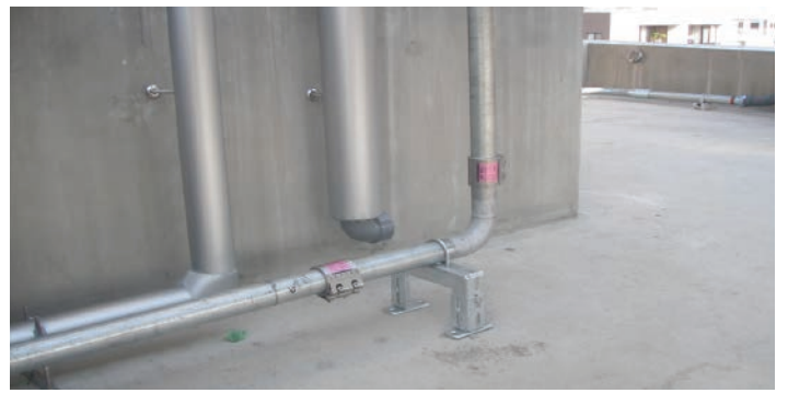
MJGF EPDM 50A, fire protection system, Japan
