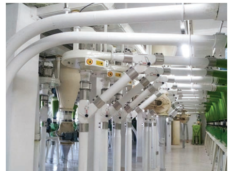
MJS EPDM + strip insert 80A~125A, wheat flour conveying system, Korea
