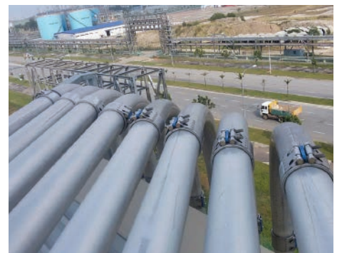
MJG, silo system.
