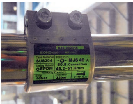
MJS EPDM 50.8mm material feeding line of injection molding system, Poland
